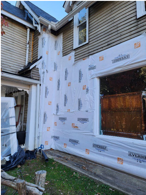
Inside corner with water filtration problem
