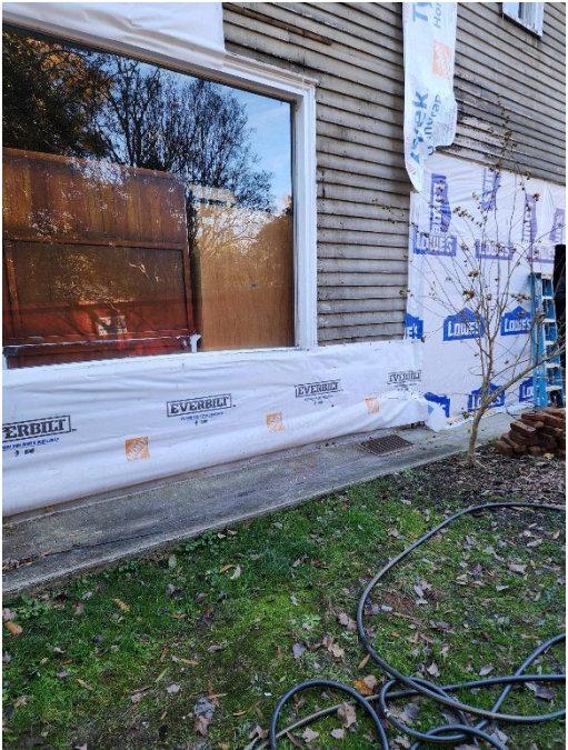
Plate glass window to be replaced with salvaged originals
